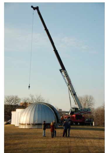
Dome removal Feb 25, 2009
